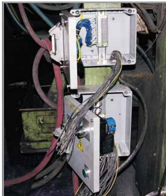
Installation of various new terminal boxes, incl. safety system.
