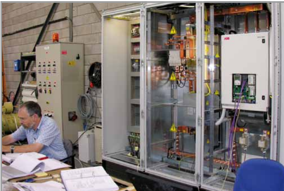
Horst Hülpsch from Hatebur knows the unspectacular-looking control cabinets inside out and is aware of their importance for flawless work with Hatebur forming machines.
