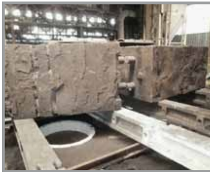
The prepared mold in the pit.
