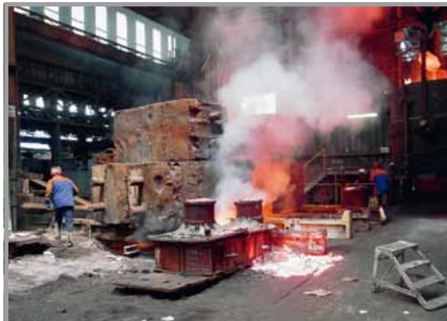
In less than ten minutes, 85 tons of liquid steel have disappeared into the earth.
