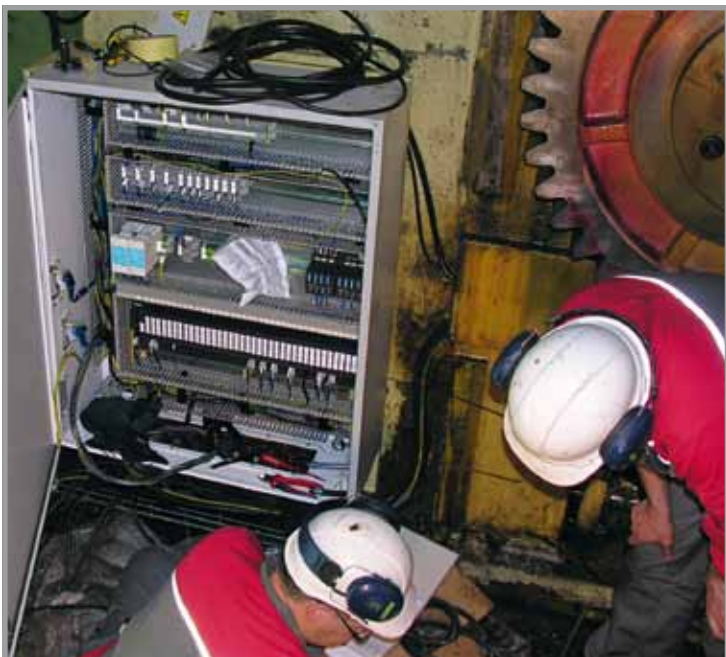
Installation and wiring on the main terminal box on the machine.
